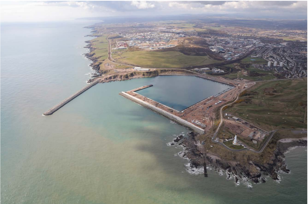
The £400 million development at Aberdeen South Harbour has been designed to accommodate larger, wider, and deeper vessels
